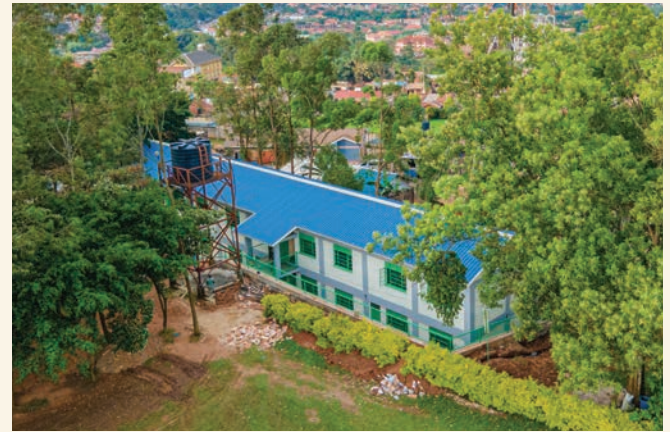
Infrastructure Capacity Development in Progress
